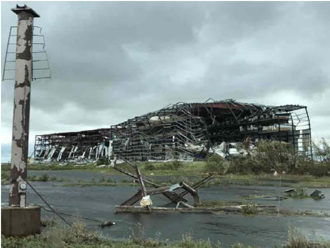
A destroyed building in Rockport, Texas (NWS)
